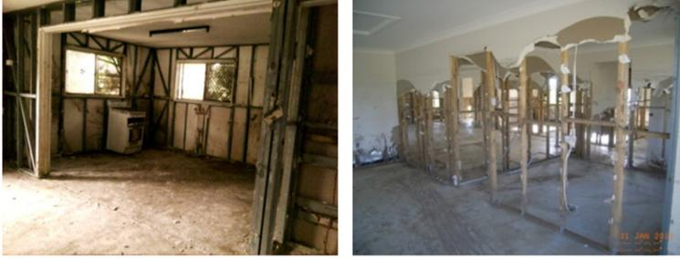
Figure 1: Examples of building damage after 2011 Queensland flooding.
