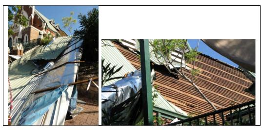
**Figure 3:** Loss of metal cladding and battens of a church. Originally a tile roof, the new metal roof was only secured to every 6<sup>th</sup> timber batten.
