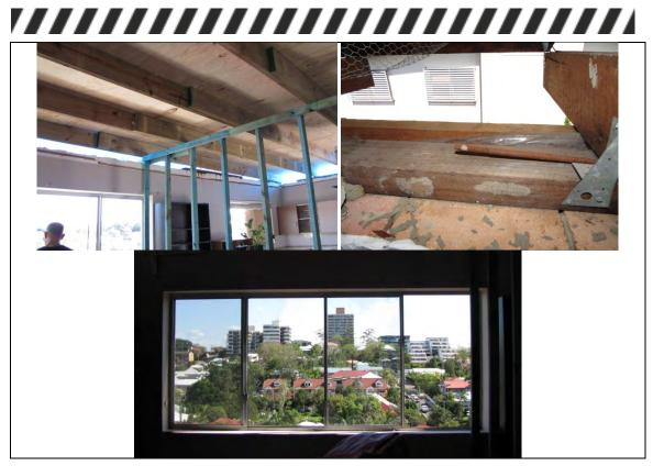
**Figure 5:** An example of complete roof loss of the top storey unit of a 3-storey apartment building (new roofing currently being installed). Original timber rafters had inadequate tie down to withstand internal pressure due to the breakage of a large southern facing window. The unit was also located on top of an escarpment (outlook shown in the lower photograph) and may have experienced slightly higher wind speeds.
