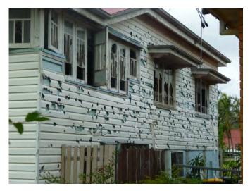
**Figure 7:** Hail damage to windows and vinyl cladding of an older house. The proximity of the neighbouring house on the right and the size of the window shades suggest hail being driven at a sharp angle by the wind.
