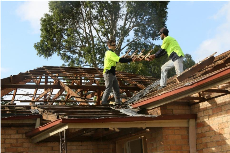
*Figure A.1 Extraction of as built batten to rafter connections*
