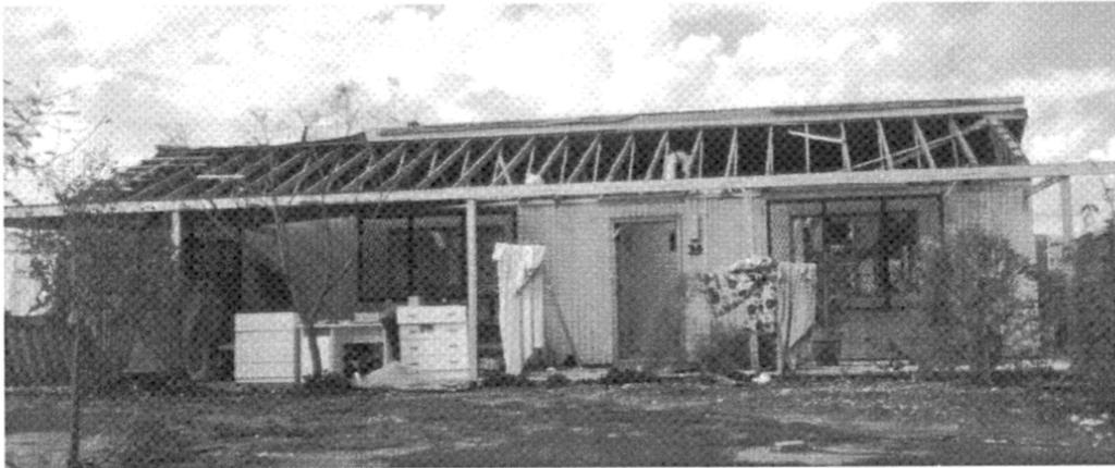
*Figure 2.3 Loss of roof cladding and battens during cyclone Vance (Reardon et al. 1999)*
