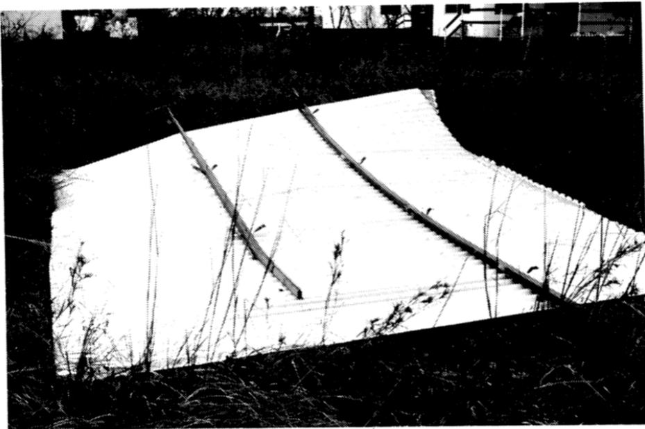
*Figure 2.1 Batten to rafter failure observed during cyclone Kathy (Boughton and Reardon 1984).*
