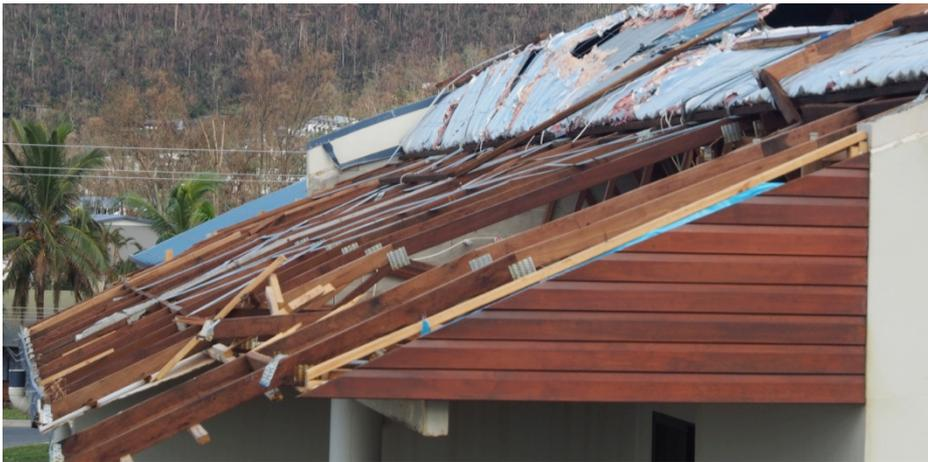
*Figure 2.5 Batten to truss connection failure in a contemporary apartment building (Boughton et al. 2017)*
