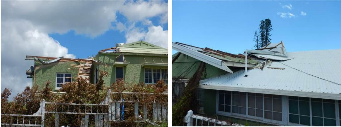
Figure 1. Wind-induced roofing failure due to poor framing connections in Yeppoon, Australia following Cyclone Marcia (2015)
