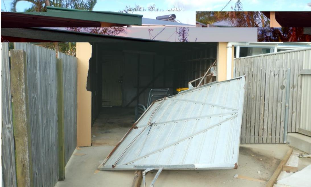
Figure 3. Wind-induced garage door failure due to poor bracing in Yeppoon, Australia following Cyclone Marcia (2015)
