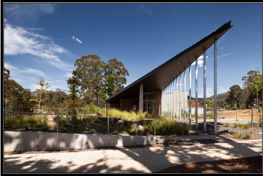
**Figure 6.15:** The new Marysville police station dominates the landscape. The veranda provides little shelter from the sun or rain, and the path has a rough stone and gravel surface that is difficult to negotiate.<sup>178</sup>
