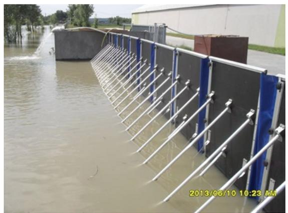
FIGURE 6: EXAMPLES OF TEMPORARY FLOOD BARRIERS (BLUEMONT, 2021)
