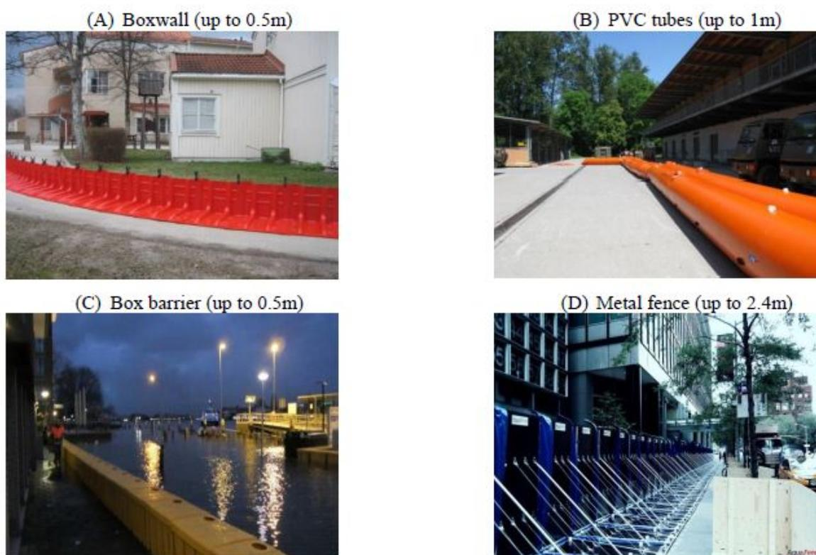
FIGURE 3: EXAMPLES OF TEMPORARY FLOOD BARRIERS (BLUEMONT, 2015)
