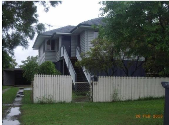
Figure 4. Examples of elevating floor levels
