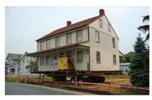
(D) Placing the structure on new foundations
