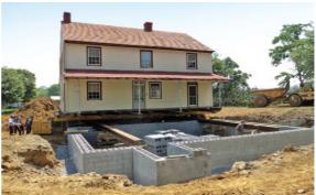
Figure 6. Relocating a structure to a new site (FEMA, 2014)
