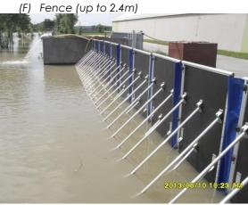
Figure 10. Examples of flood barriers (Bluemont, 2015)
