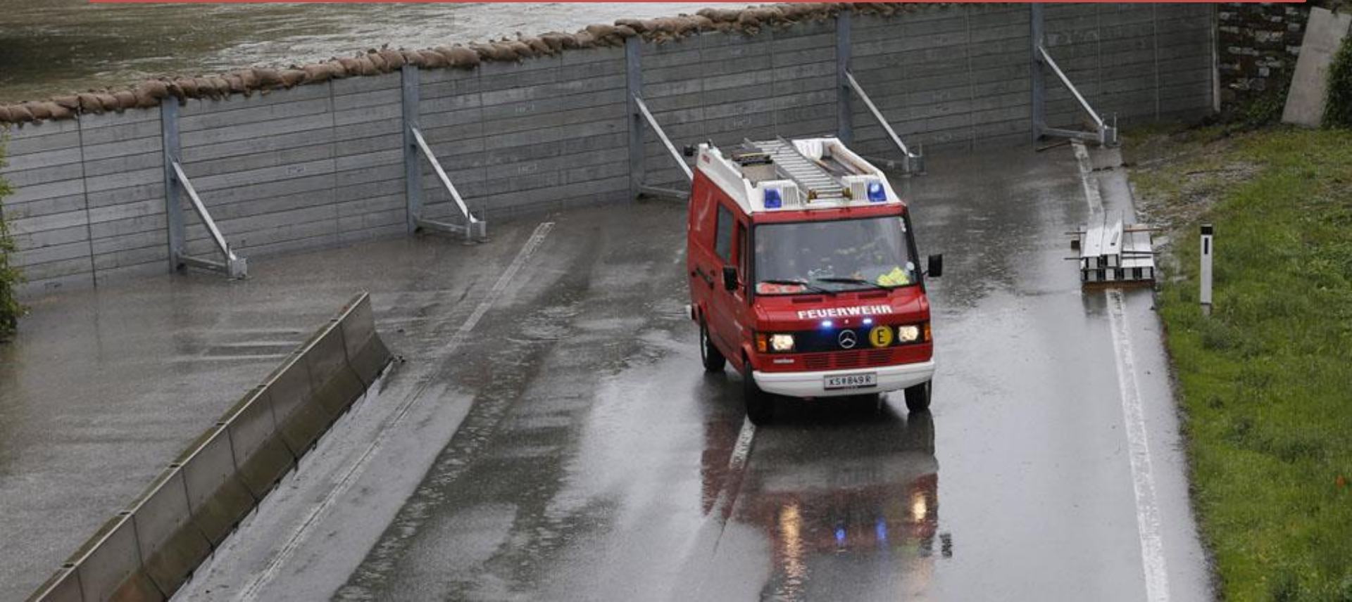
Danube River flood barrier, 2013
