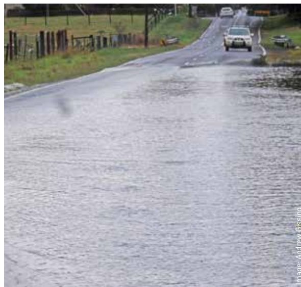
The research location included a local road closed by floodwaters. There were no depth markers or side railings along the section of flooded road.
