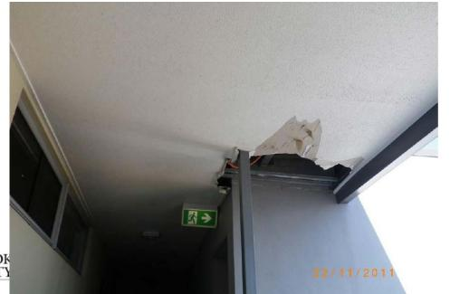
Inadequate box gutters for roof area. No overflow outlets for when over-capacity or when wind driven leaf litter is blocking down pipe.
