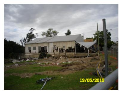
Figure 4.9 Site of House 6 with very little remaining. Evidently a timber framed house on brick piers. Note scour on downstream side of Dowling Street exposing in-ground services. Tyre business premises in background.
