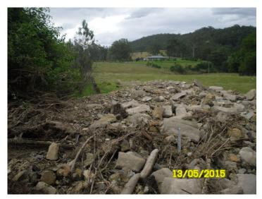
Figure 4.23 Myall Creek bridge. Eroded debris from northern abutment deposited immediately downstream. The northern approach embankment is behind shrubbery at left of image.
