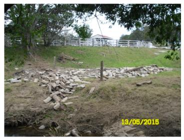
Figure 4.25 Myall Creek bridge. Eroded debris from southern abutment deposited immediately downstream of bridge.
