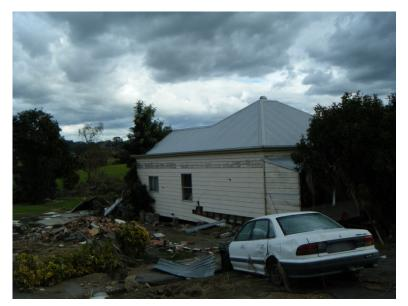
Figure 4.7 House 4. Note that house has been moved off its supporting timber stumps. The peak water level is estimated to have been 3.5m above ground level at this location (approximately gutter level on the house).
