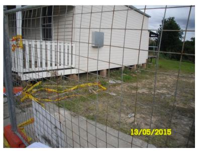
Figure 4.4 House 1, north elevation. Note ant-caps in foreground and displaced brick piers at right hand side of veranda and at rear corner of house.
