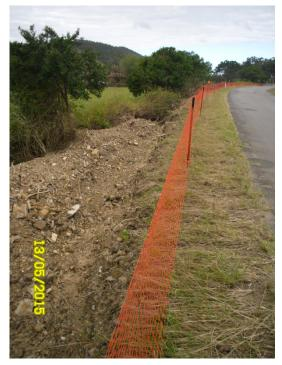
Figure 4.21 Myall Creek bridge, northern approach embankment. Flattened grass and severe scour on downstream side of embankment indicative of over-topping. Southern end of bridge visible in top right of image.
