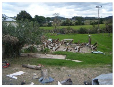
Figure 4.8 Site of House 5. Evidently a timber framed house on timber stumps. Piers are estimated to be 250mm diameter with 600 mm embedment and approximately 1.5 m projection above ground.
