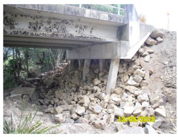
Figure 4.22 Myall Creek bridge. Repaired northern abutment.
