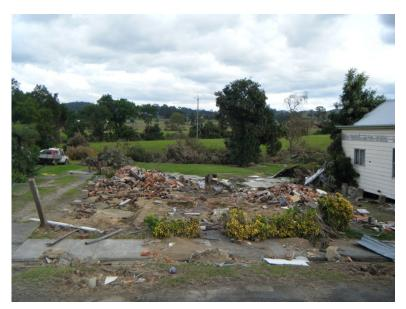
Figure 4.6 Site of House 3. Evidently a timber framed house on brick piers.
