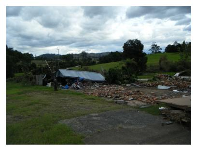
Figure 4.5 Site of House 2. Evidently a timber framed house on brick piers.
