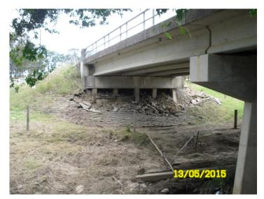
Figure 4.24 Myall Creek bridge. Scour damage to southern abutment.
