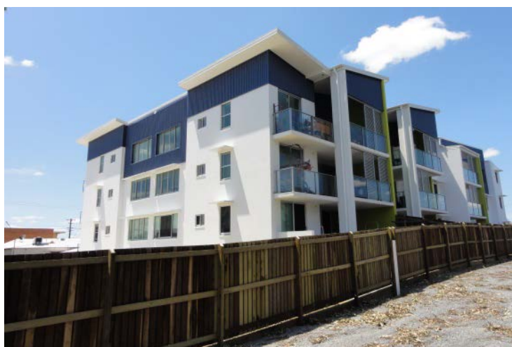
Figure 8: A new apartment building in a storm-affected neighbourhood. All windows on the exposed southern side were undamaged, indicating the improved performance of new window glass.
