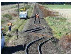
Figure 1: Canterbury earthquake 2010. Buckling of train tracks near Rolleston, New Zealand (Source: Dr Dave Petley).
