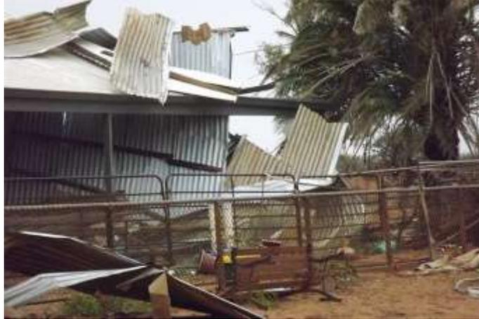
**Figure 15.** Roof loss at truss/batten connection Boolathana Carnarvon (Courtesy: Mary Bettini)
