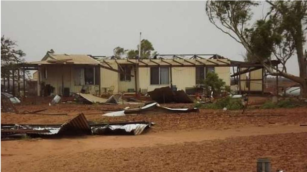
**Figure 14.** Roof loss at batten-to-truss connection in Carnarvon (Courtesy: Mary Bettini)
