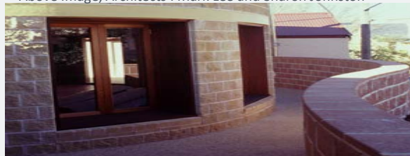
Curved non combustible walls with recessed windows preferably metal and sliding doors which can be enclosed by protective bushfire shutters. Above Image, Architects : Cracknell & Lonergan
