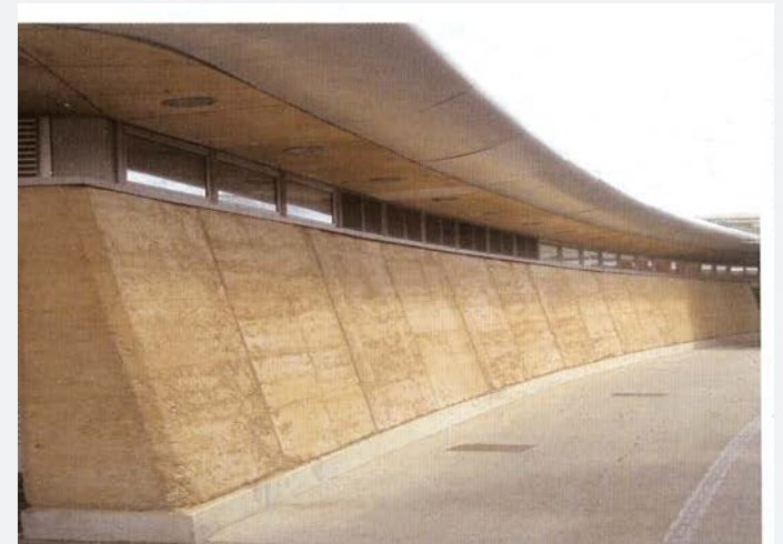
Small windows with protective overhang placed at the wall and roof junction, on the side facing a bushfire threat, reduces both potential ember entry and earthquake damage while encouraging greater internal air flow. Image from: Walker, P. (2005). Rammed earth : design and construction guidelines
