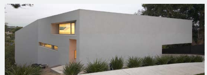
Wall facing anticipated bushfire threat direction constructed of non combustible materials with no or limited glazing. Adjoining wall with recessed door and windows and inbuilt bushfire shutters. Architects: Johnston Marklee & Associates
