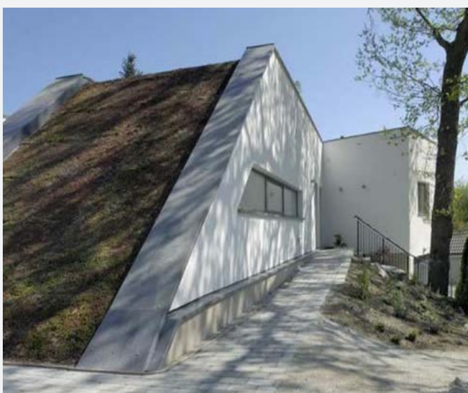
Angled earth covered roof encourages bushfires to move over and away from house. Architects: RB Arkitektur Image from: http://www.google.com.au/imgres?imgurl=http://www.trendir.com/house-design/underground-home-designs-swiss-mountain-house
