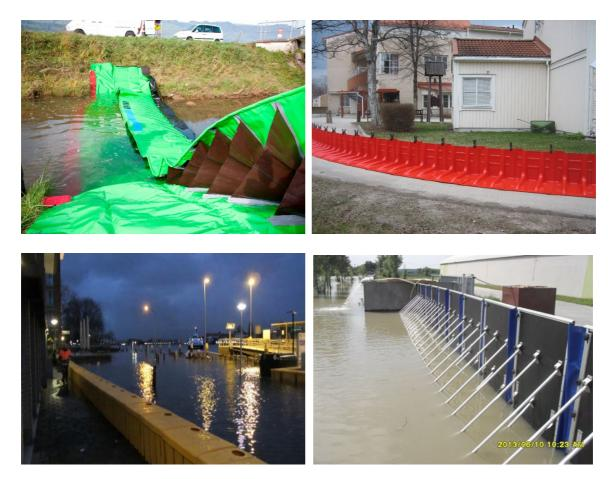
FIGURE 6: EXAMPLES OF TEMPORARY FLOOD BARRIERS (BLUEMONT, 2021)
