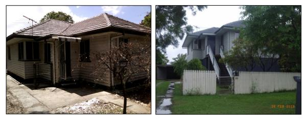
FIGURE 3: AUSTRALIAN EXAMPLE OF MITIGATION THROUGH ELEVATION
