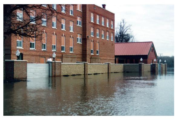
FIGURE 5: AN EXAMPLE OF A FLOODWALL (FEMA, 2013)
