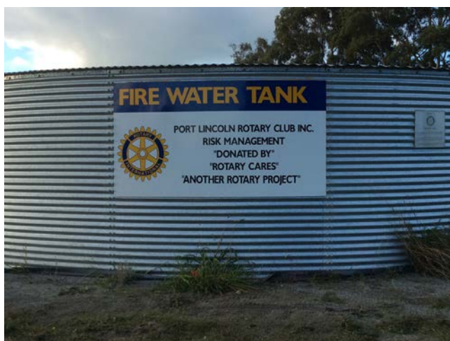
Community fire water tanks around Lake Eyre Peninsula are a constant reminder to people that the threat of fire is ever present.
