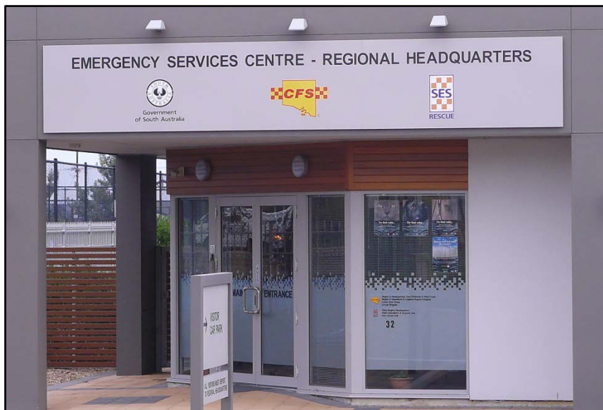
Illustration 5: South Australia Police (SAPOL) station, Liverpool Street, Port Lincoln (top) and the Emergency Services Centre, Matthew Place, Port Lincoln. SAPOL, the Country Fire Service (CFS) and the State Emergency Service (SES) all participated in research interviews or focus groups.
