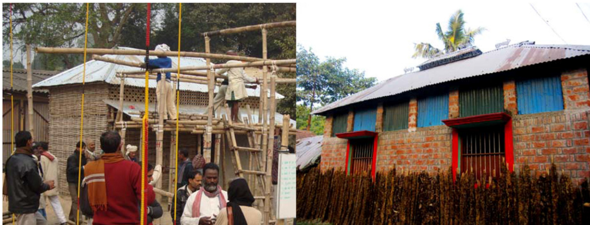
Fig. 4. Reconstruction in Bihar, in 2008, using bamboo (left) (source — SEEDS) and in 2014 using brick (right).
