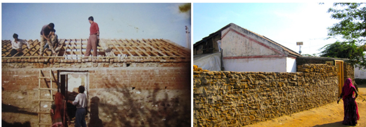
Fig. 3. Reconstruction in Patanka, Gujarat, in 2001 (left) (source — SEEDS); houses in 2015 (right).
