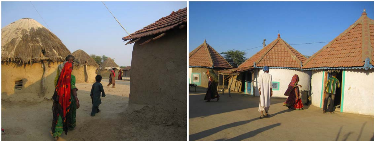
Figure 3: Photos of traditional mud houses in Hodko, Gujarat, prior to the 2001 earthquake (left) and after reconstruction (right) (source: author)
