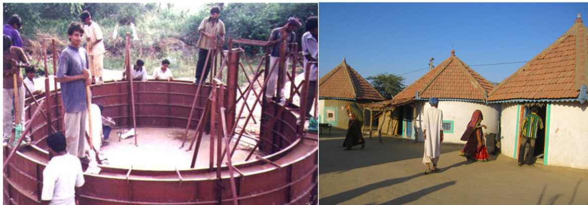
Fig. 2. Reconstruction in Hodko, Gujarat, in 2001 (left) (source- Hunnarshala); Houses in 2015 (right).
