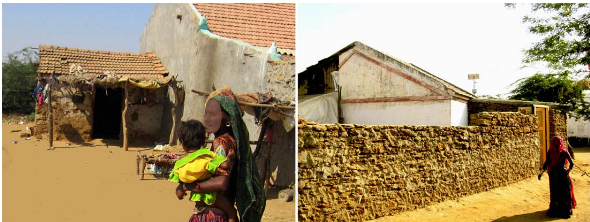
Figure 4: Photos of traditional uncoarsed stone masonry houses in Patanka, Gujarat, prior to the 2001 earthquake (left) and after the reconstruction (right) (source: author)
