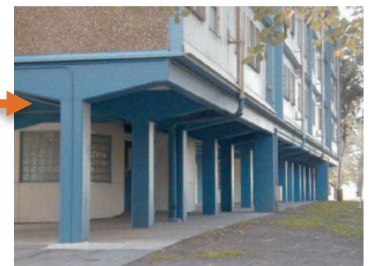
Figure 2: Soft storey building 1 . Menegon et al. (2019)
