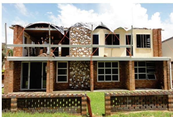
Internal Pressure Damage
