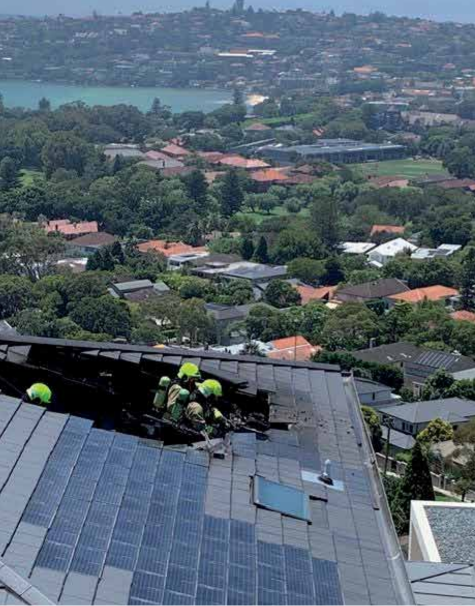
Working amongst a damaged and live solar tile array is a potentially fatal exercise for fire and emergency service crews.
