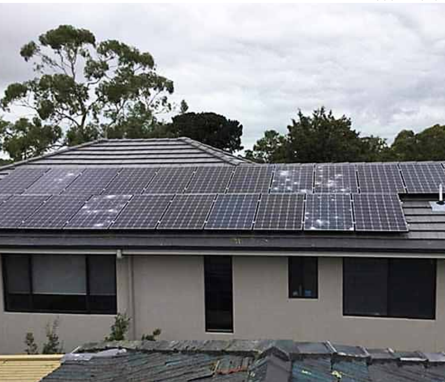
Above: Solar panels damaged by hail pose a safety risk to fire and emergency personnel.
