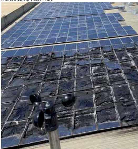
Hail damage to a solar panel array of a Moorebank, NSW factory sparked a significant roof fire at the property.
