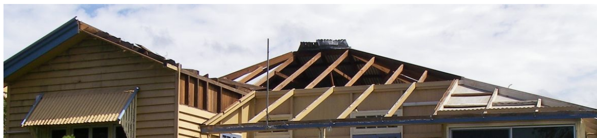
FIGURE 1. REMOVAL OF ROOF CLADDING AND BATTENS FROM WINDWARD FACE
