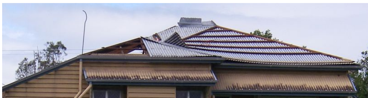
FIGURE 2. PART OF THE ROOF CLADDING WITH BATTENS STILL ATTACHED FLIPPED ON TO LEEWARD SIDE
