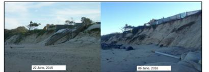
Dune erosion at Old Bar Beach (NSW) showing further retreat and damage resulting from a storm surge on 5 May 2016 (Photo credit: M. Griffiths, MidCoast Council, NSW)
